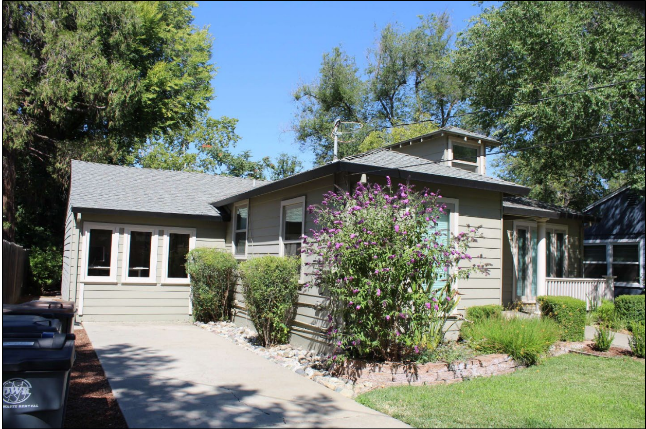
Photo 4 of 15: East and south facades, looking northwest
