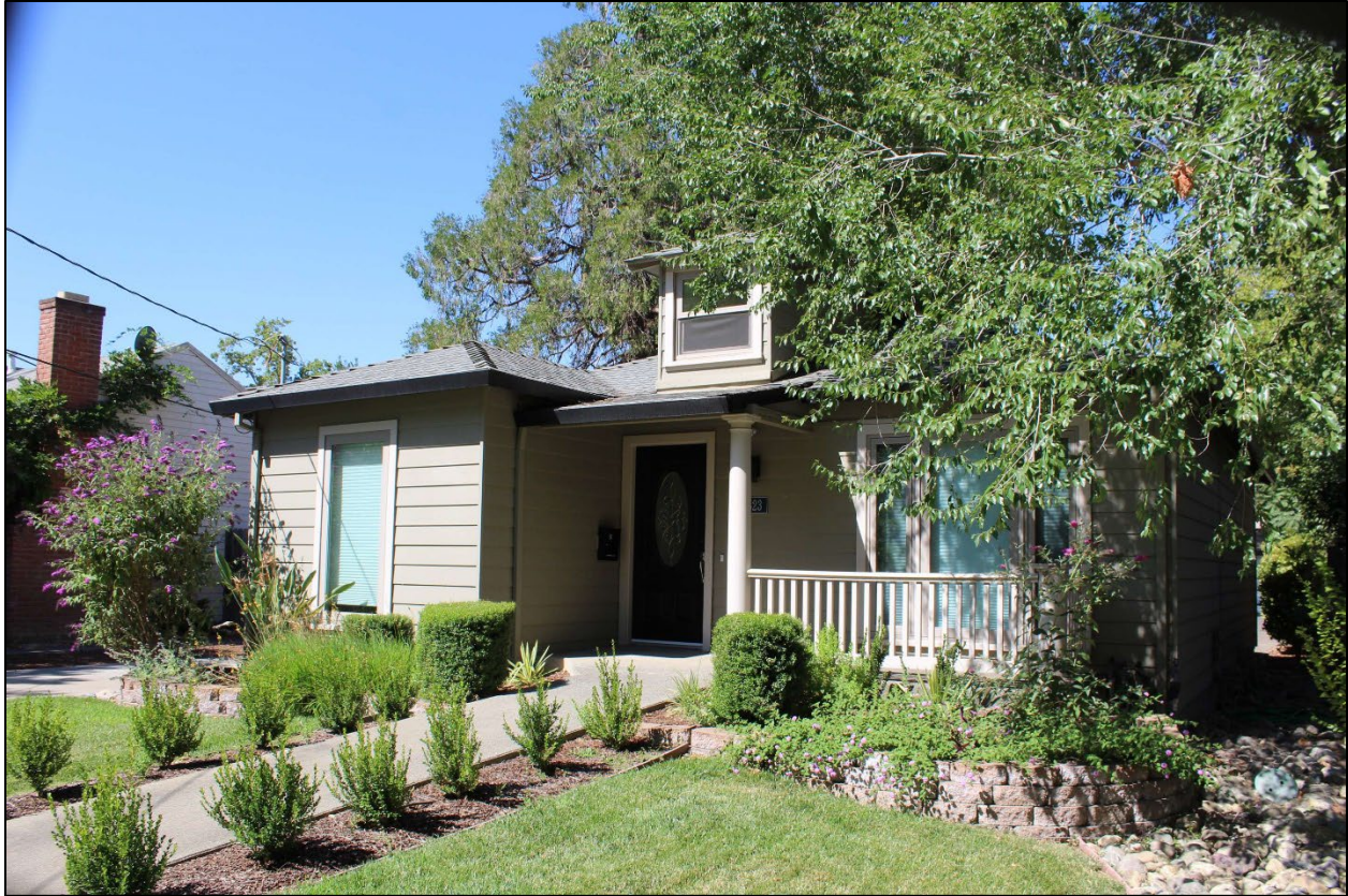
Photo 2 of 15: Front (west) façade, looking southwest
