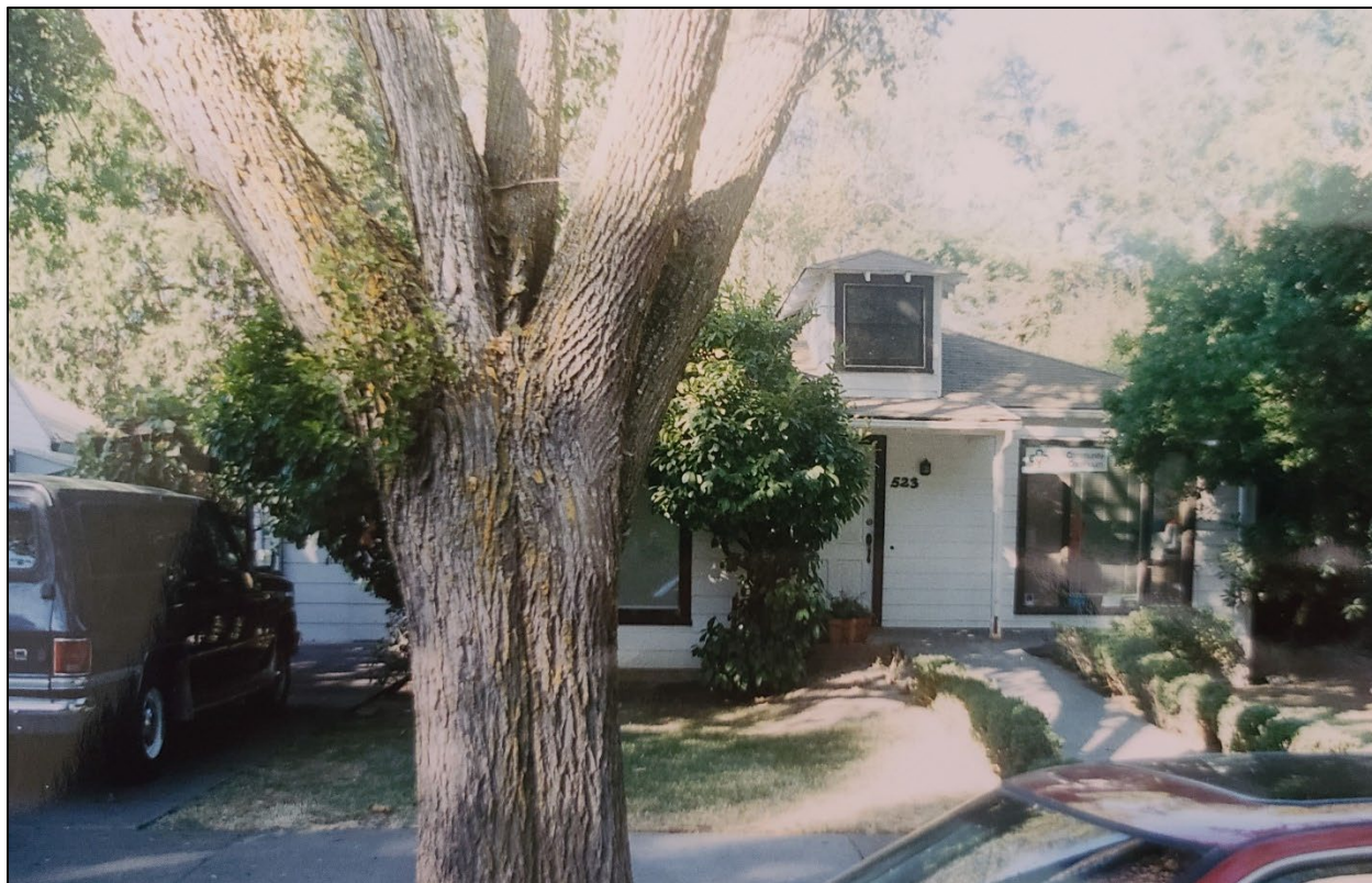
Figure 10: Building at 523 G Street photographed circa 1997
