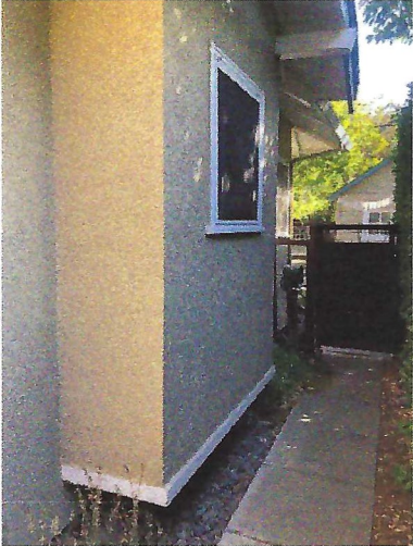
To address sagging issues, footings to be added to support pop-out section of bathroom
