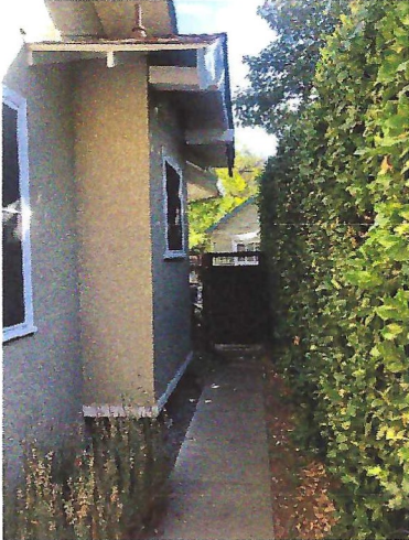
To address sagging issues, footings to be added to support pop-out section of bathroom
